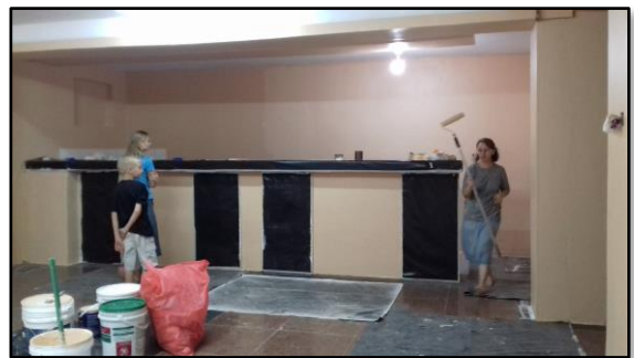
DURING: Back of Main Room
