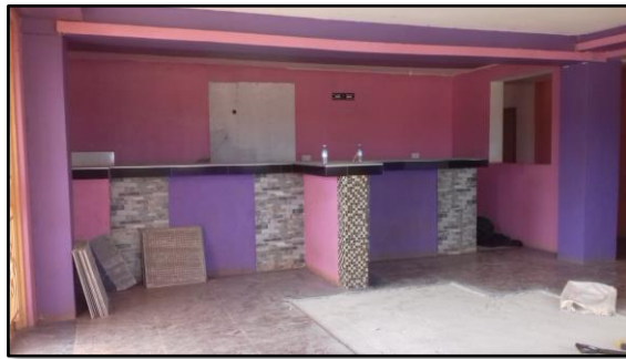
BEFORE: Back of Main Room (Tile repairs in progress.)
